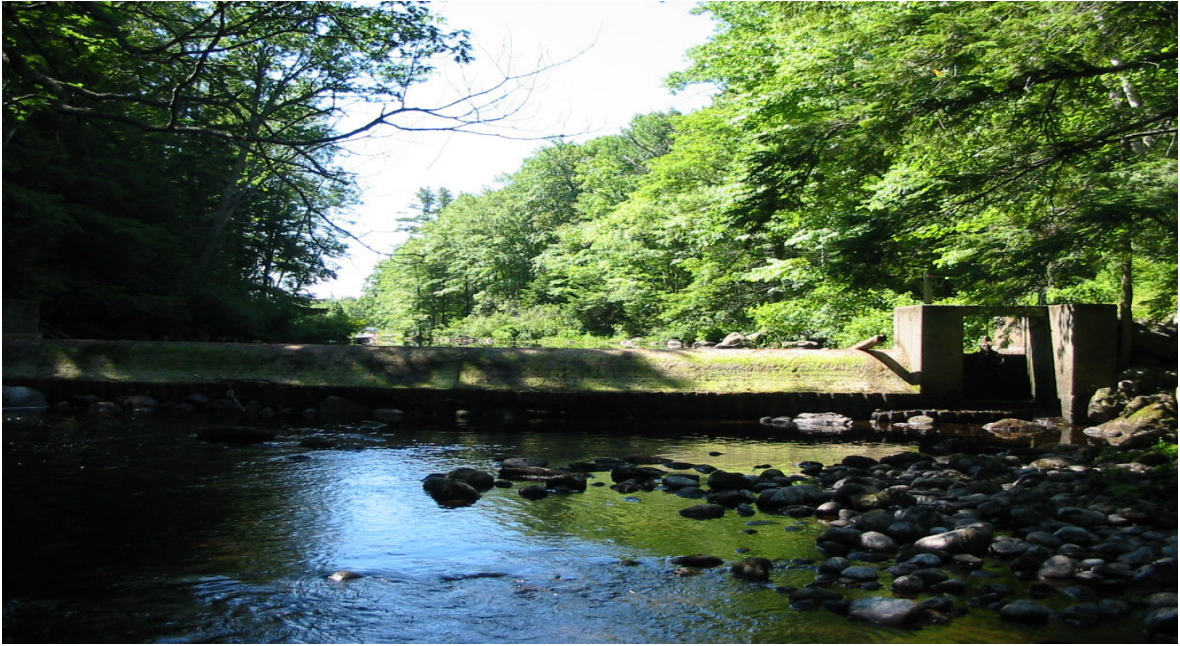
Sheepscot Lake Dam; July 2003
