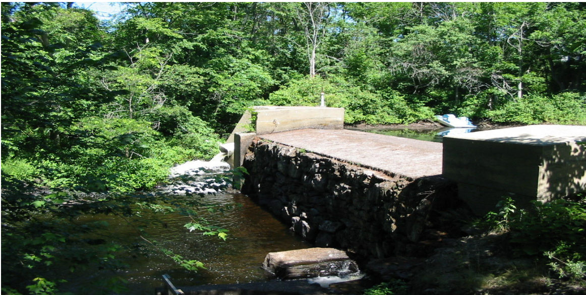
Coopers Mills Dam; July 2003
